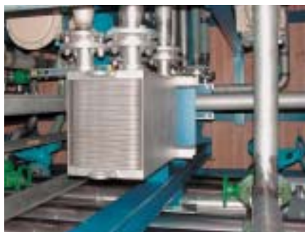
SIGMAWIG ST 12 tempering of chemical reactor thermoil/ ethylenglycol
