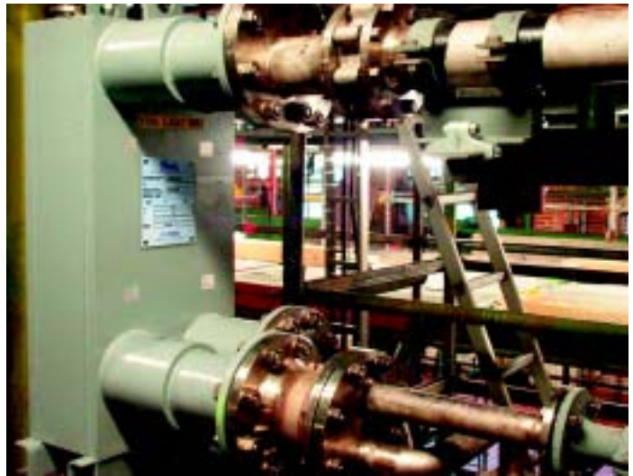
SIGMAWIG ST 30 for steam condensation
